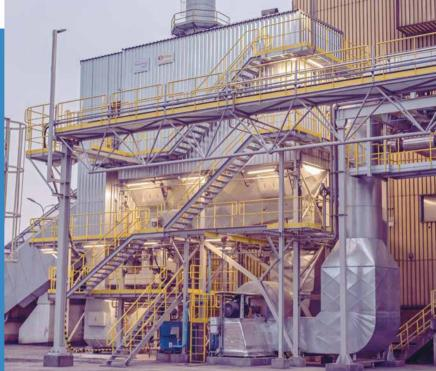
Application of technology with mechanical reactor gives the opportunity to design the installation with much smaller dimensions. This reduces the investment costs and allows to adjust a new installation in place of the existing one.
